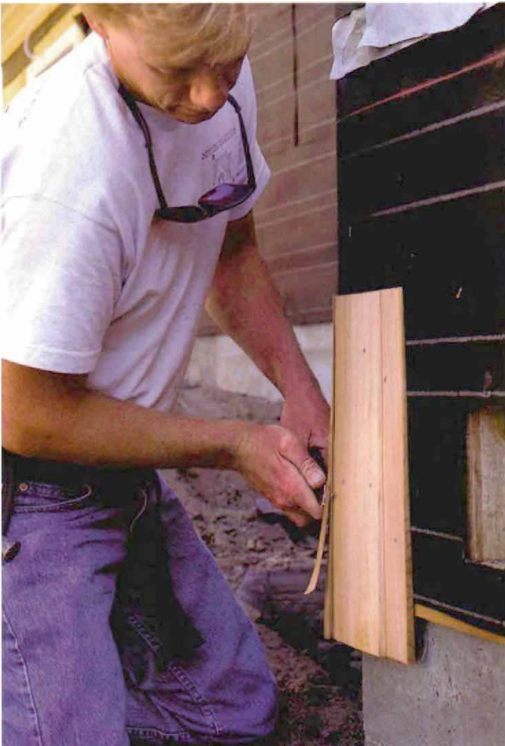
After the corners are built, fill in the field. A level can be used to mark the layout when the distance between corners is short; otherwise, a chalkline works well.
